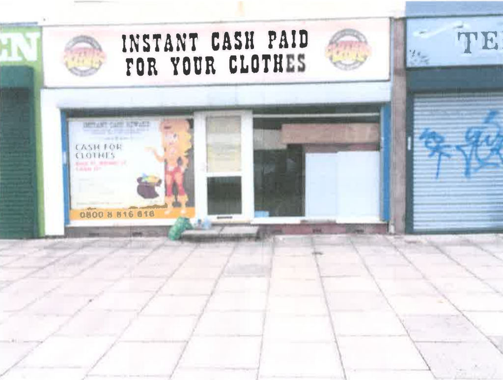
View of premises from pavement
